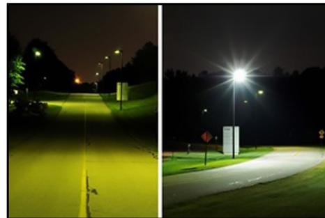
*Current lighting, left, will be replaced by LED fixtures, right, increasing visibility, saving on cost, and reducing environmental impact. (Photo courtesy of Kyle Hawkins)*
